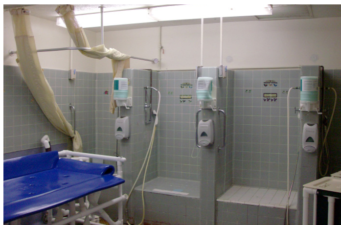
Old shower stalls in the HMC Long Term Care facility.
