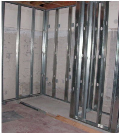
Construction is underway! The shower stalls have been torn out and the framework laid for the new stalls.
